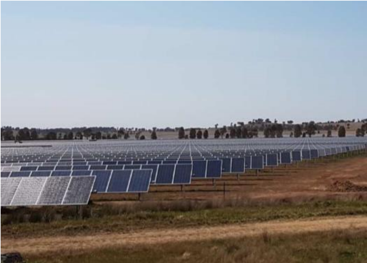
Installation of last Modules –
