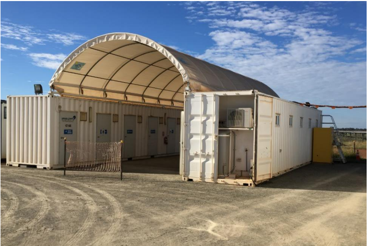
O&M Building Set up
