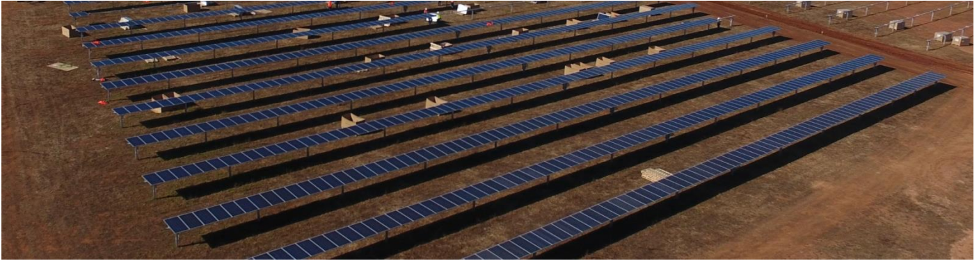
First Panels installed
