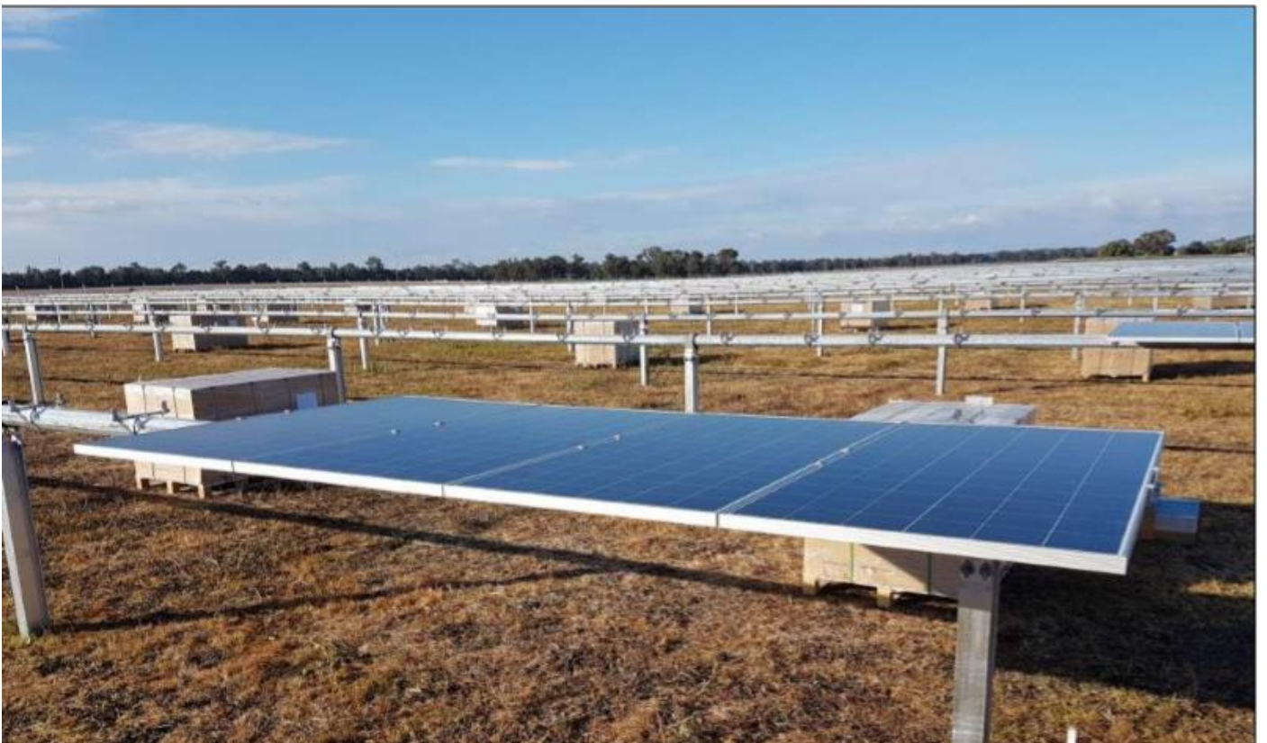
First Modules Installed
