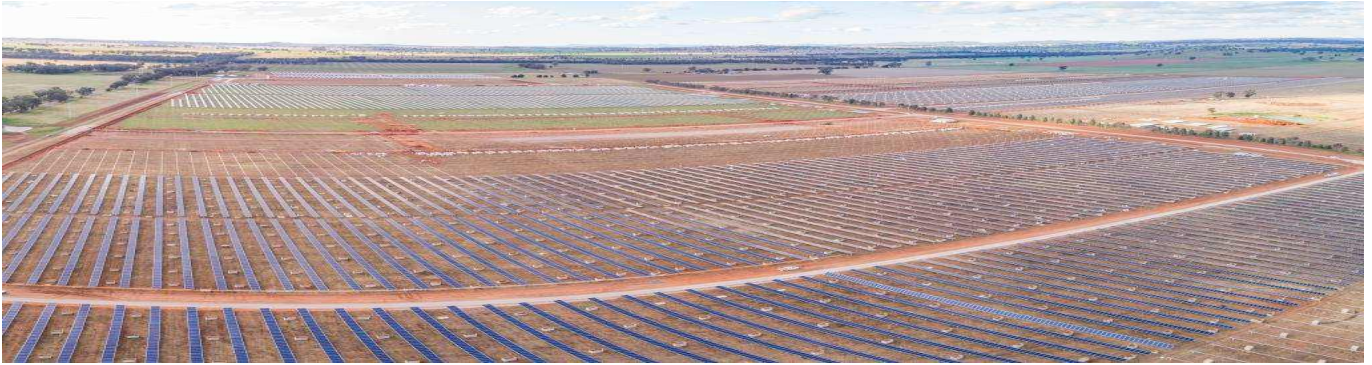
First Panels installed
