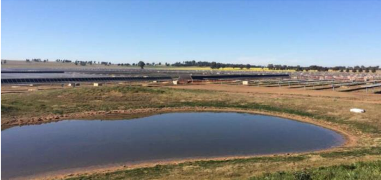
Installation of Modules – Last area zone E
