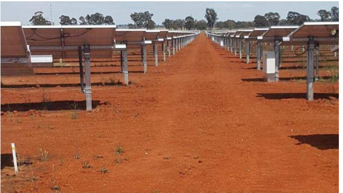
Internal Road Conformation
