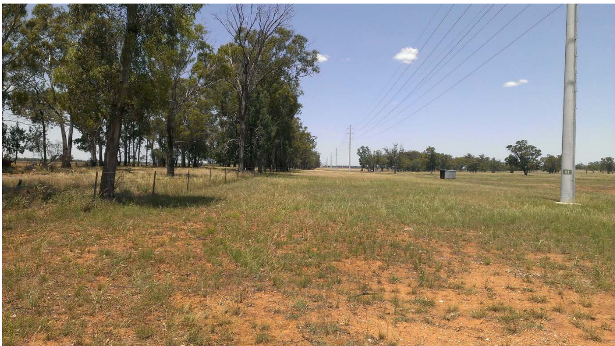
Figure 3-6 View of proposed above ground transmission line route, to the west of Pat Meredith Drive
