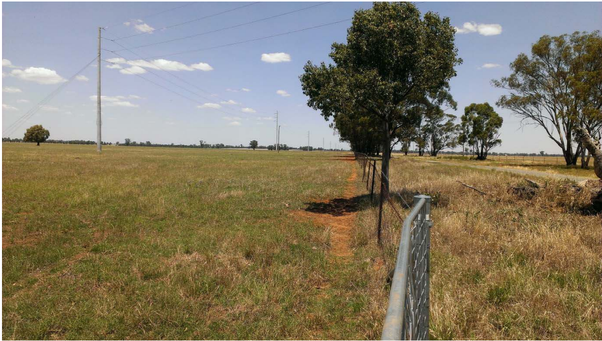
Figure 3-5 View of 132/66 kv power line near western boundary of proposal site and Pat Meredith Drive
