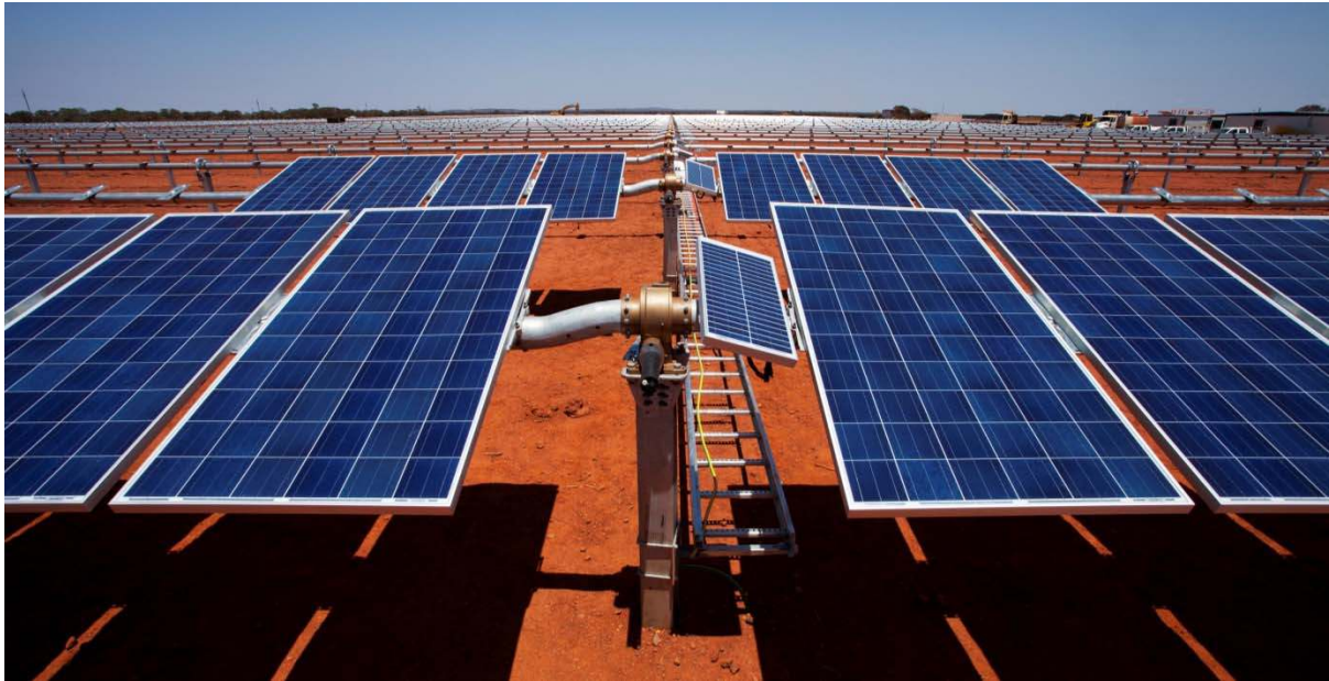
Figure 3-10 Example of a single-axis mounting system after panel installation
