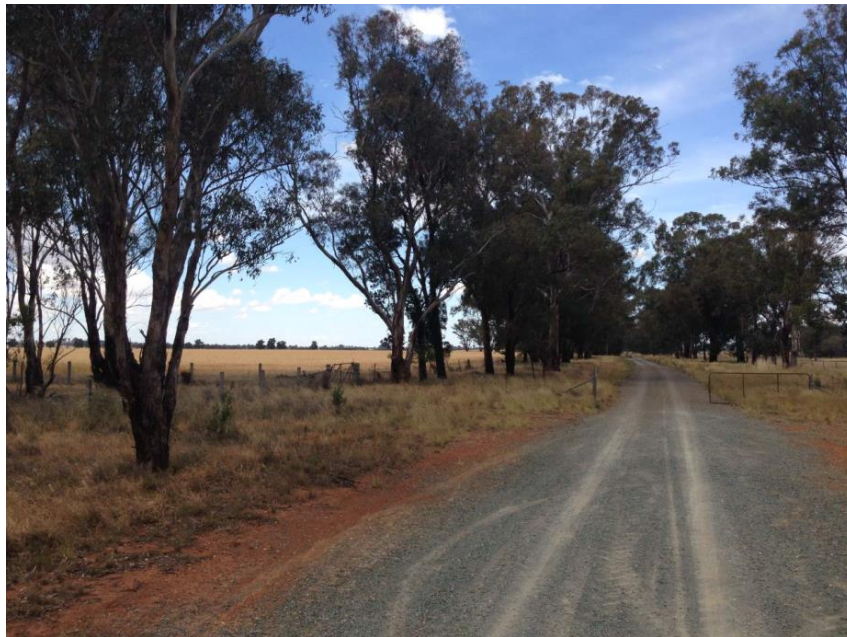
Figure 1 : Pat Meredith Drive (access road for the project)
